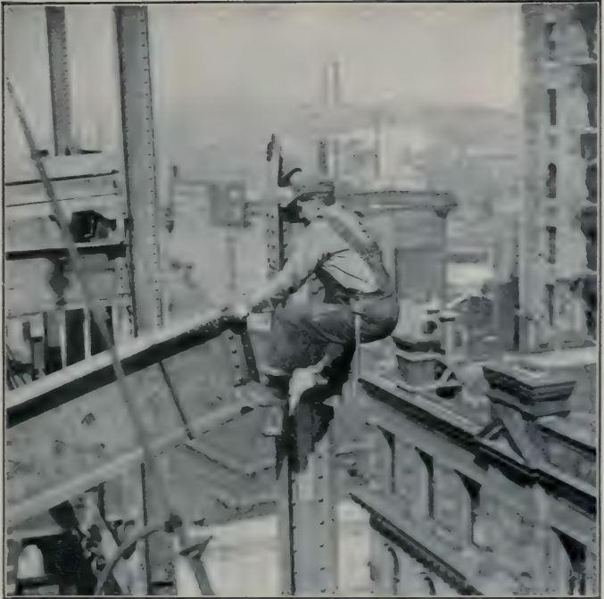
STRUCTURAL STEEL WORK ON A MODERN SKYSCRAPER
